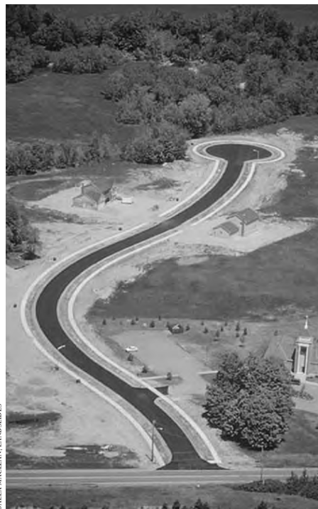
This cul-de-sac serving a small subdivision is wider than the state highway it connects to.
